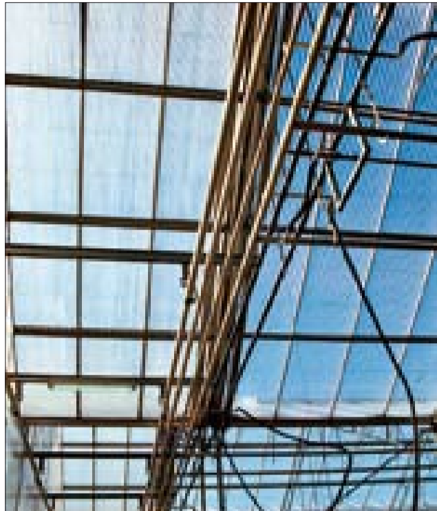
Visible quality: on the left, conventional polycarbonate double-skin sheets showing pronounced signs of weathering that let in less sunlight. Right: clear view with PLEXIGLAS ALLTOP® double-skin sheets.
